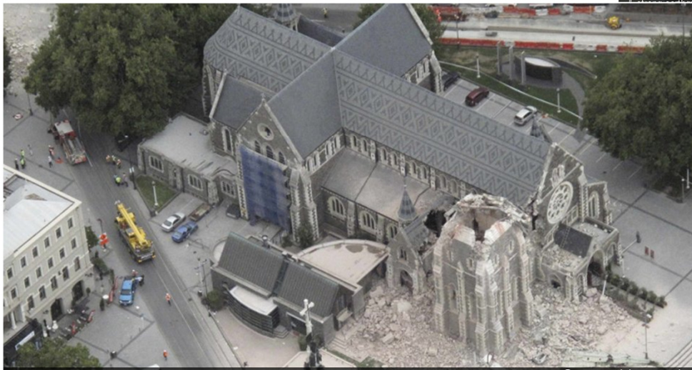
The earthquake also dealt severe damage to the famous Christchurch Cathedral. Its spire toppled into the square below.
